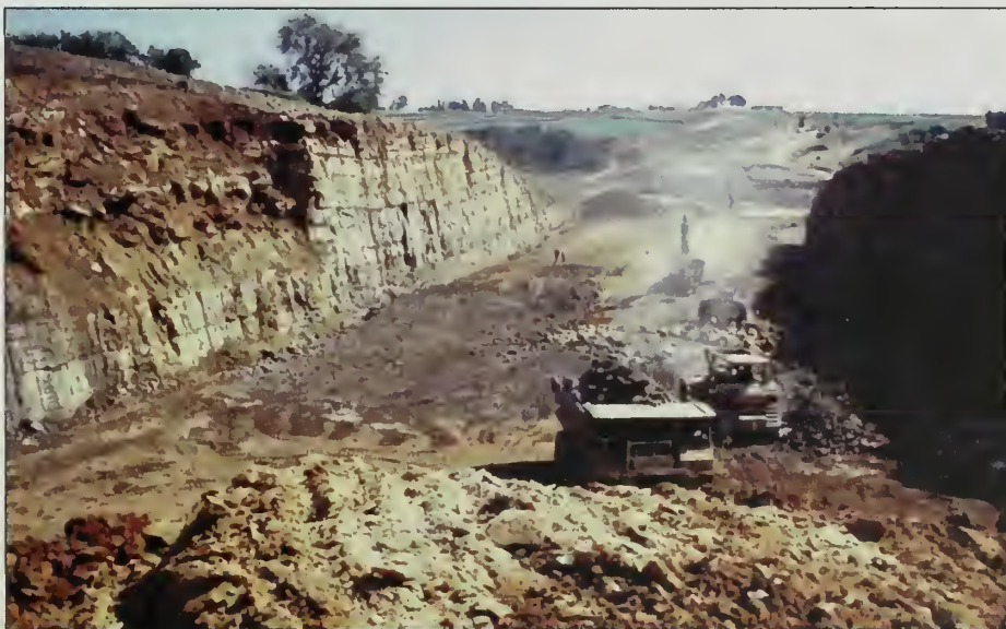
Figure 11 U.S. Highway 151 fairgrounds road cut under construction in 2001.
